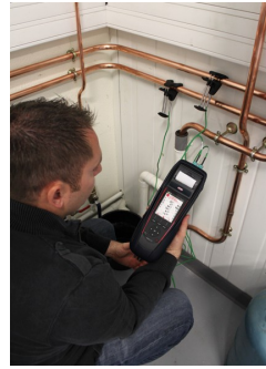
DHW network temperature
